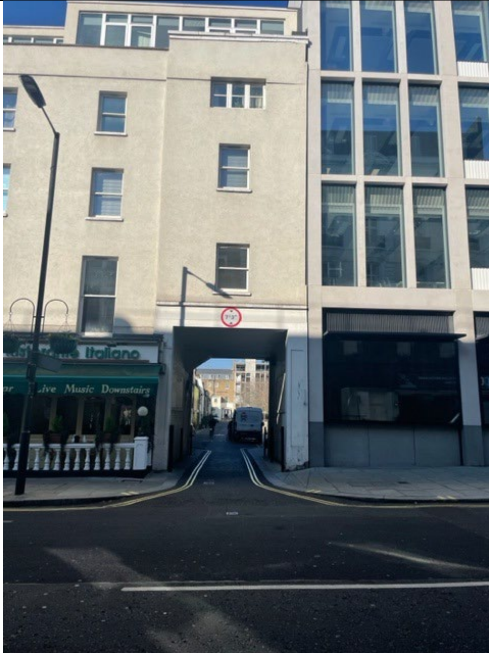
Vehicular Access Via Arch (another Arch at the northern end of the Mews) from Craven Road to Chilworth Mews, which leads to the off street loading bay for 50 Eastbourne Terrace.
